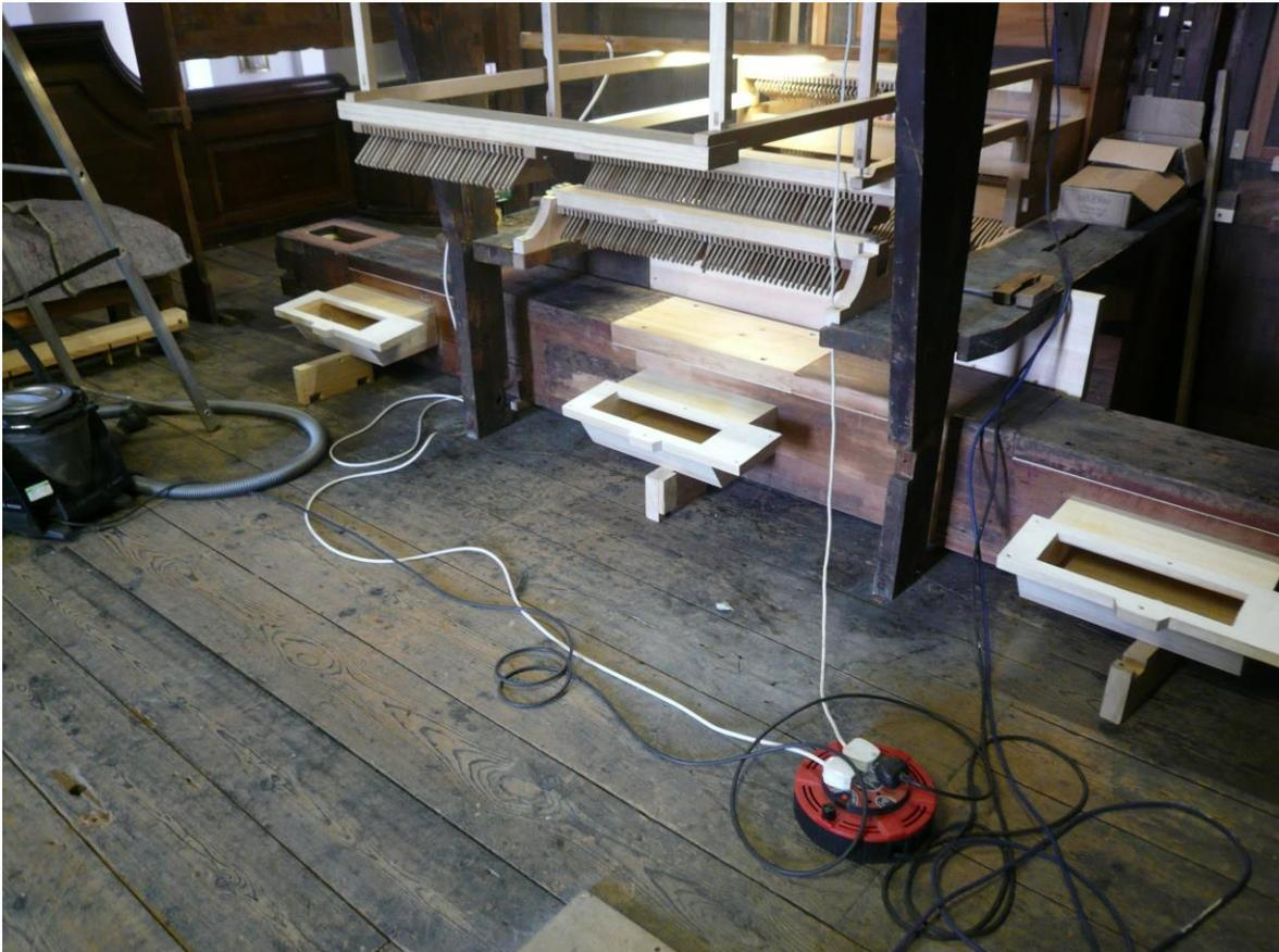
The Swell trunk was reconstructed with an internal cross section of 134 x 60mm after the size of a blocked up hole which was discovered in the Bass face-board of the Great wind box.
