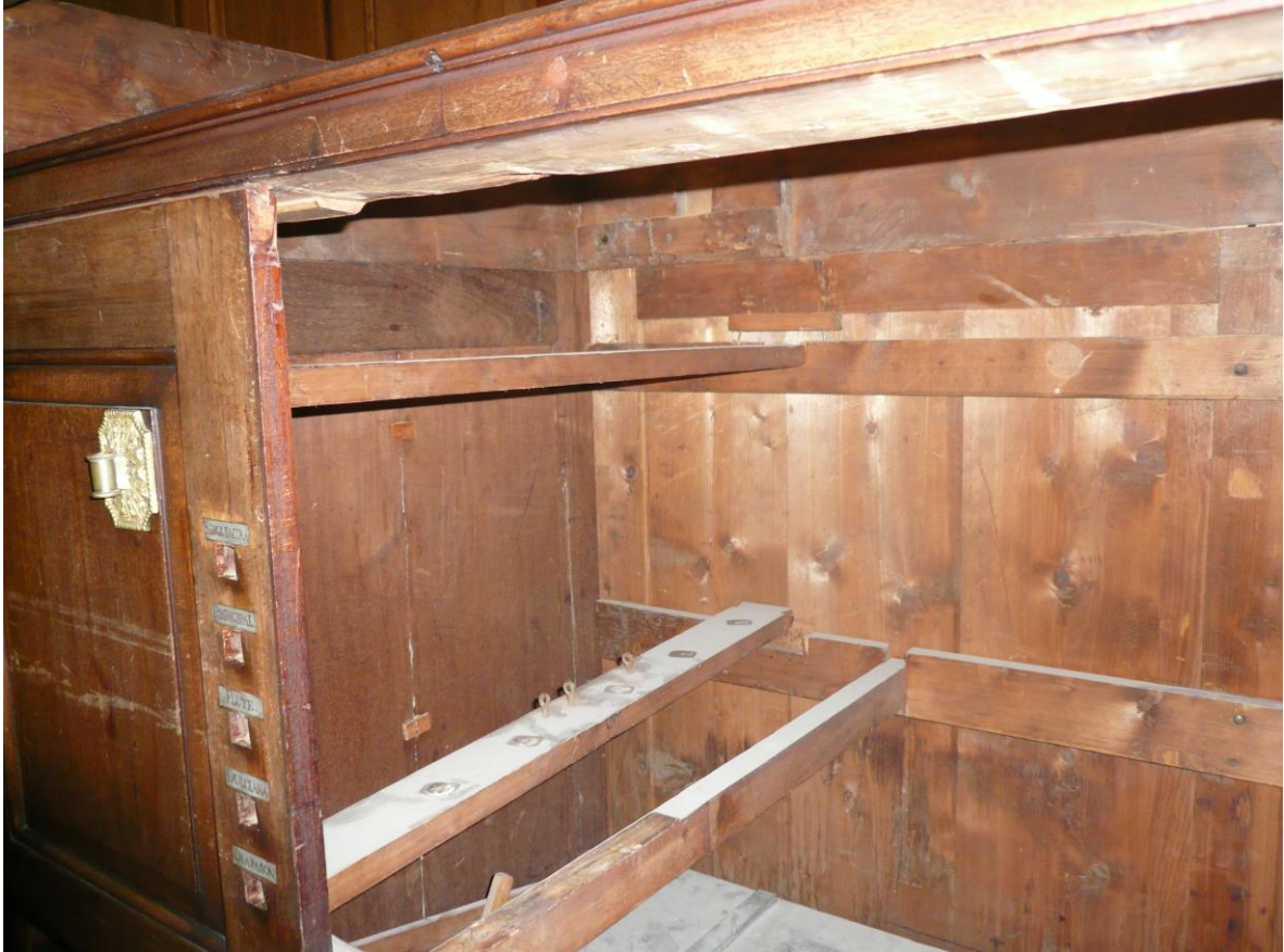
Condition of the finish during dismantling
